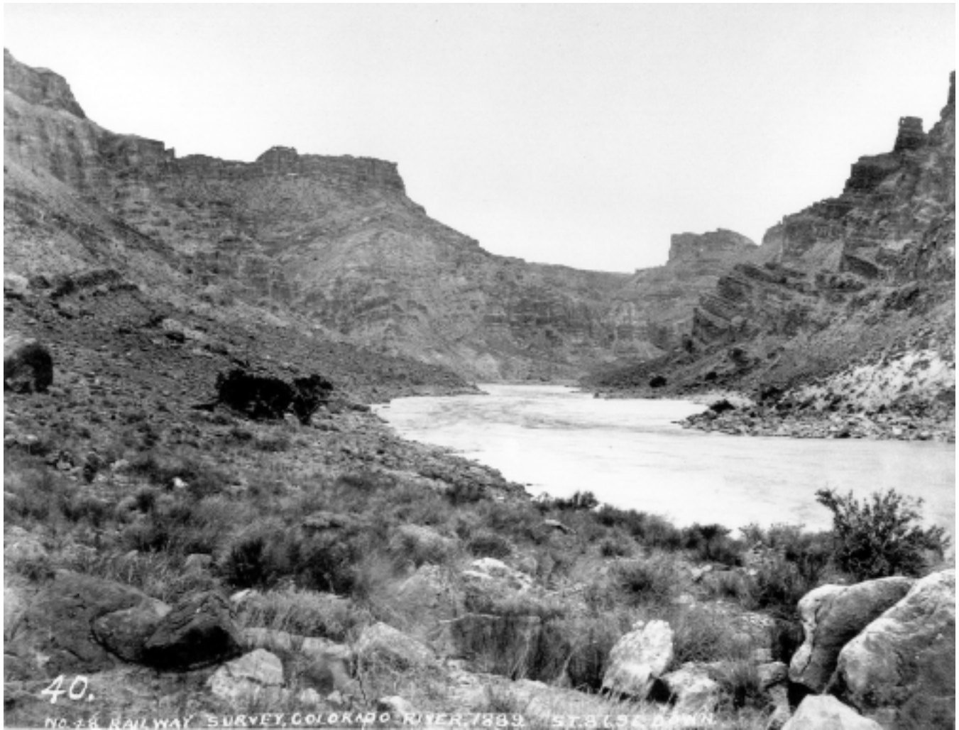
Figure 1. Rapid 1 from River Left. (files s2908-1889.tif and s2908-1994.tif)
